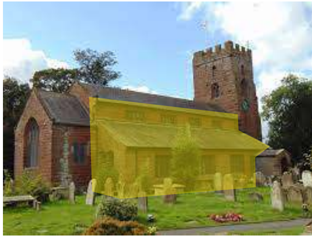
EXTENT OF EXTERNAL SCAFFOLDING & HOARDING
