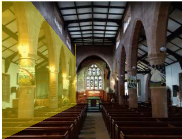
EXTENT OF INTERNAL SCAFFOLDING
